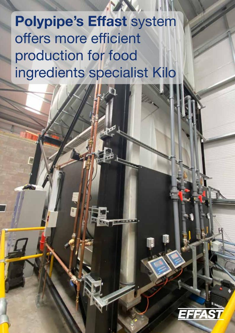
Polypipe's Effast ABS products provide a robust, lightweight system that reduces pressure loss. The pipe and fitting systems offer a safe and secure choice for chilled or potable water, food stuffs and beverage applications in a commercial environment.
